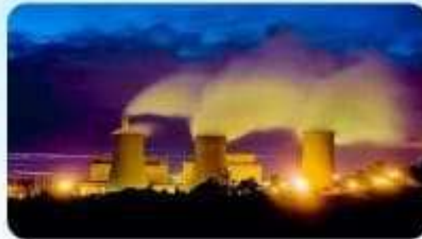
Fossil fuel power plant
