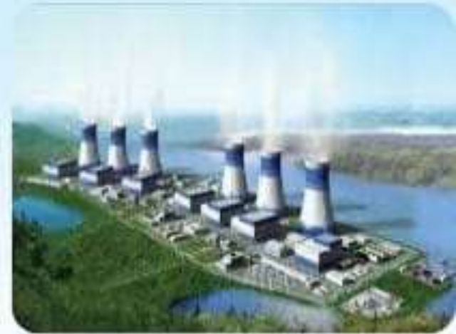
Nuclear power plant
